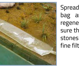
Spread out the fine filter bag and place it in the regeneration zone. Make sure that there are no sharp stones or objects under the fine filter bag.
