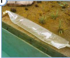
Spread out the fine filter bag and place it in the regeneration zone. Make sure that there are no sharp stones or objects under the fine filter bag.
